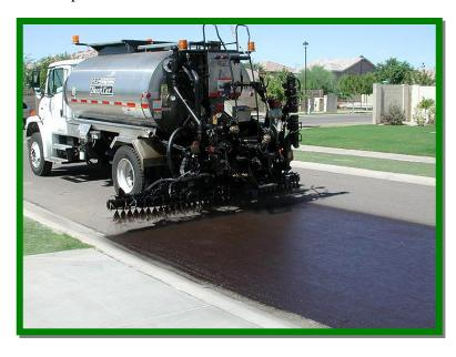
Stone Lock Fog Seal is a quick set light texture (QSLT) material consisting of a base, hard pen asphalt emulsion which is further prepared for resistance to environmental & chemical destruction through the interfusing of NEOS<sup>TM</sup> bio-resin modified ground tire rubber. Upon application the Stone Lock Fog Seal penetrates deep into tiny fissures and asphalt voids rejuvenating and flexibilizing the uppermost region of aged and embrittled asphalt.
